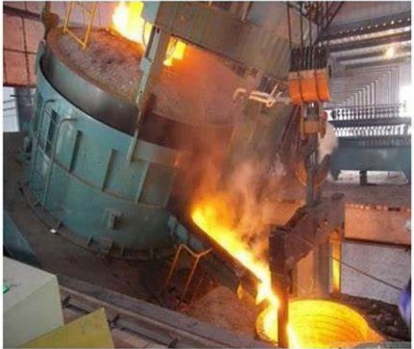
Photo Caption: Submerged Arc Furnaces (output ~4–6 MW), commonly used for the production of ferrosilicon and ferromanganese. Advantages include high energy efficiency and productivity.
